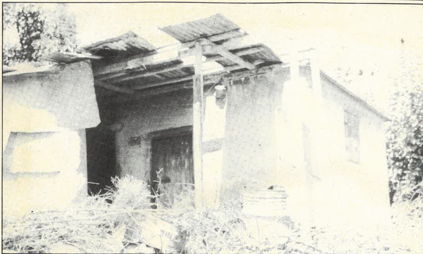
● Most of the inhabitants of Dheisheh live in UN-built relief shelters — this one houses a family of 20
