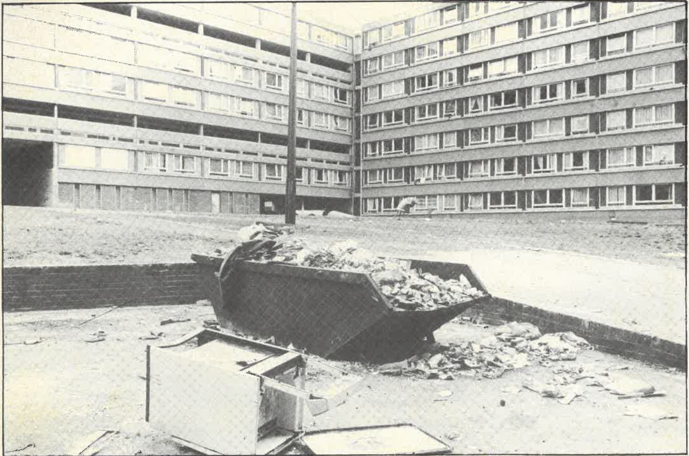
● The failure by the Housing Executive to provide adequate waste disposal facilities has led to some tenants having to burn their rubbish to stem the plague of rats which infests Divis
