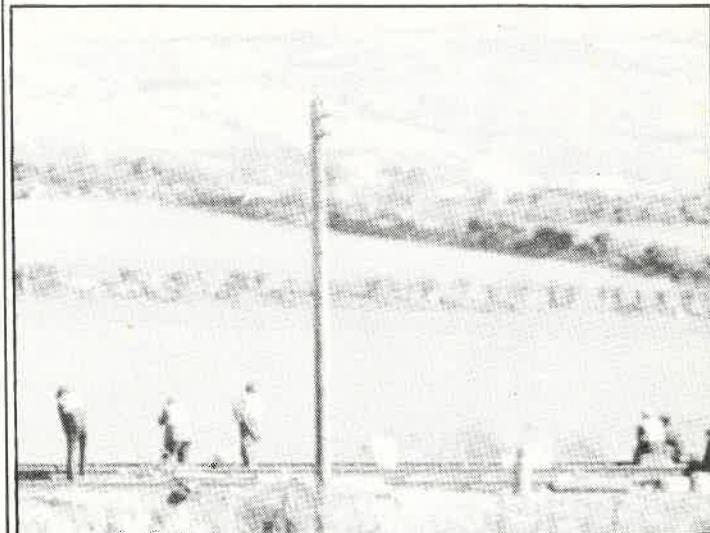
● Work begins (once again!) on repairing the Belfast-Dublin rail-link severed by IRA engineers
