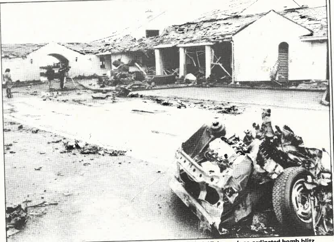
● This hotel in Campsie, County Derry, was extensively damaged in February's co-ordinated bomb blitz
